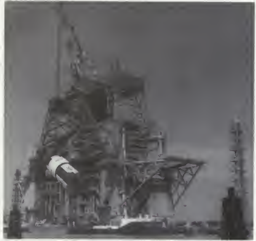
Left, an aerial view of NASA's Michoud Operations. Below, the 124-meter-tall test stand at the Mississippi Test Facility is hoisting the first operational S-IC first stage for the Saturn V into test position. Bottom, the map shows the acoustic effects of an S-IC firing.
